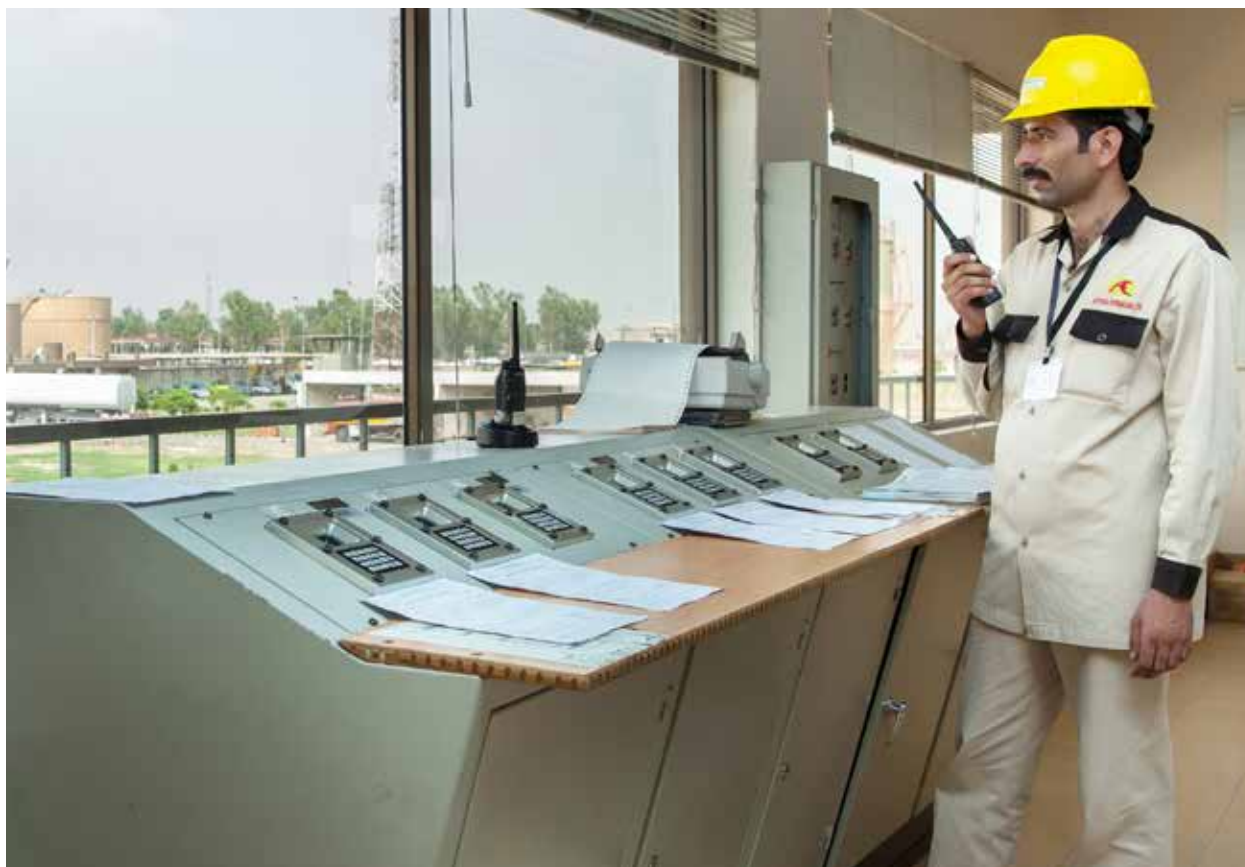
Operations Control Room
