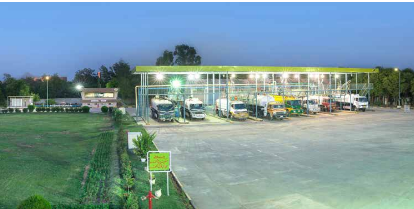
Rawalpindi Bulk Oil Terminal, Morgah
